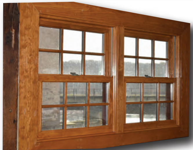
Delaware and Raritan Canal Commission headquarters, Stockton. Photos: Erica Vavrence
